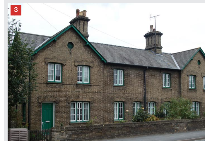
Gault brickwork in flemish bond
