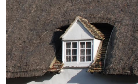
Dormer windows (plain tile dormer and later lead box)
