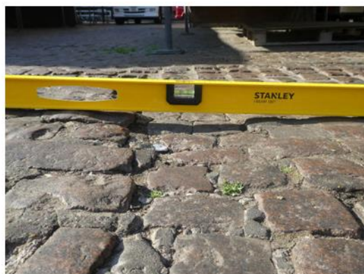
Photo 19: Zone 11 showing significant hazard and rounded/damage setts.
