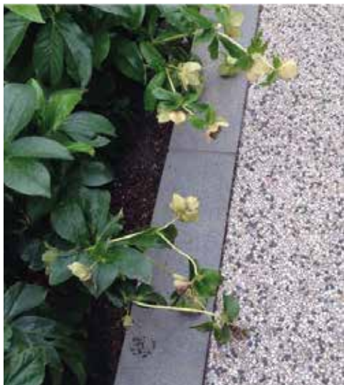
High contrast paving edges using "accent" material
