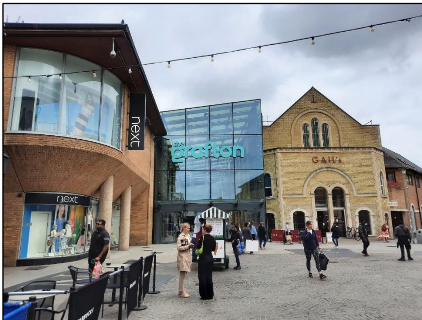
Figure 3.1: Photograph of the Grafton Centre
