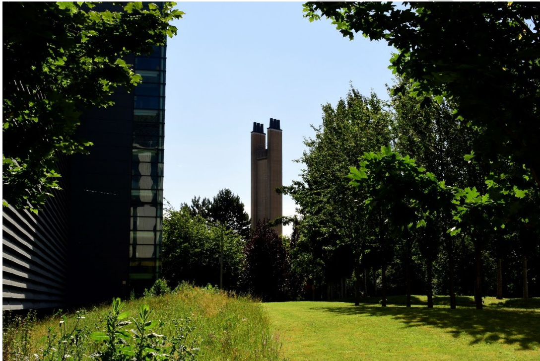
Image 5: Addenbrooke's Hospital incinerator chimney
