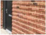
2: Example of protruding brick banding entrance areas.
