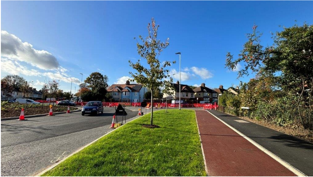
Roundabout NW quadrant
