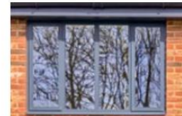
Aluminium frame - Dark grey colour to match existing bi-folding door
