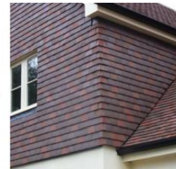
Vertical tile hanging - tile to match existing roof
