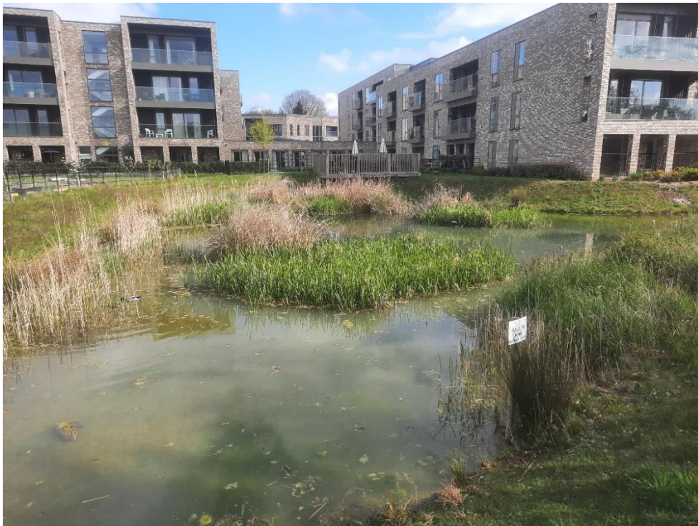
Figure 11 SuDS feature in a new development
