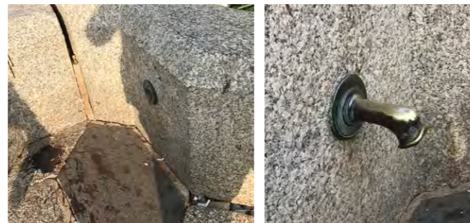
Fountain water supply existing features
