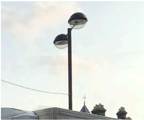
Existing lighting columns
