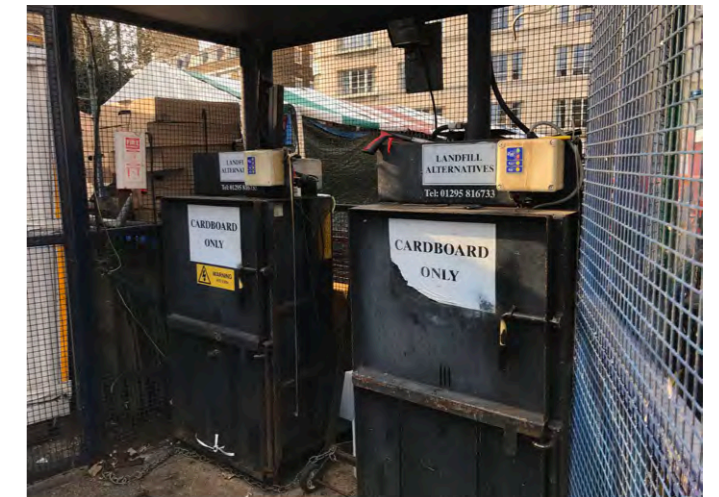
Cardboard waste compressor
