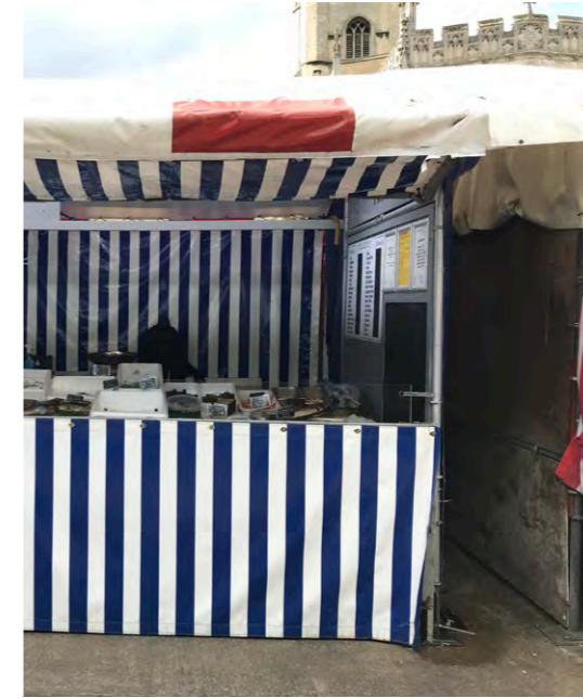
Photo showing existing drain used by fish monger for their waste
