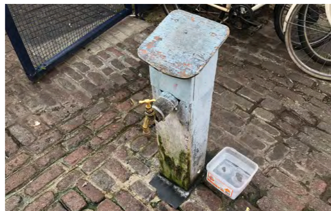
Existing water tap
