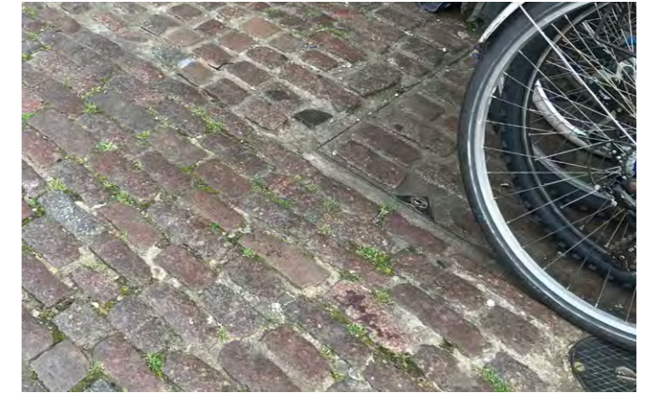
Existing recessed cover within setts
