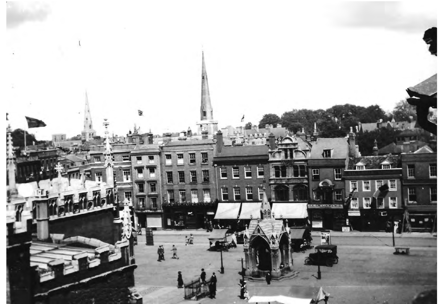
Photo from early C20 – note the original fountain design, the surface change over the now-extant underground lavatories and the lamp posts without lanterns.
