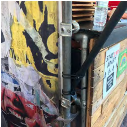
Evidence of existing Kee Klamp use by the traders
