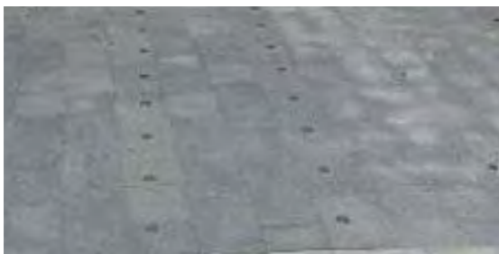
Example demarcation studs for inset parking bays
