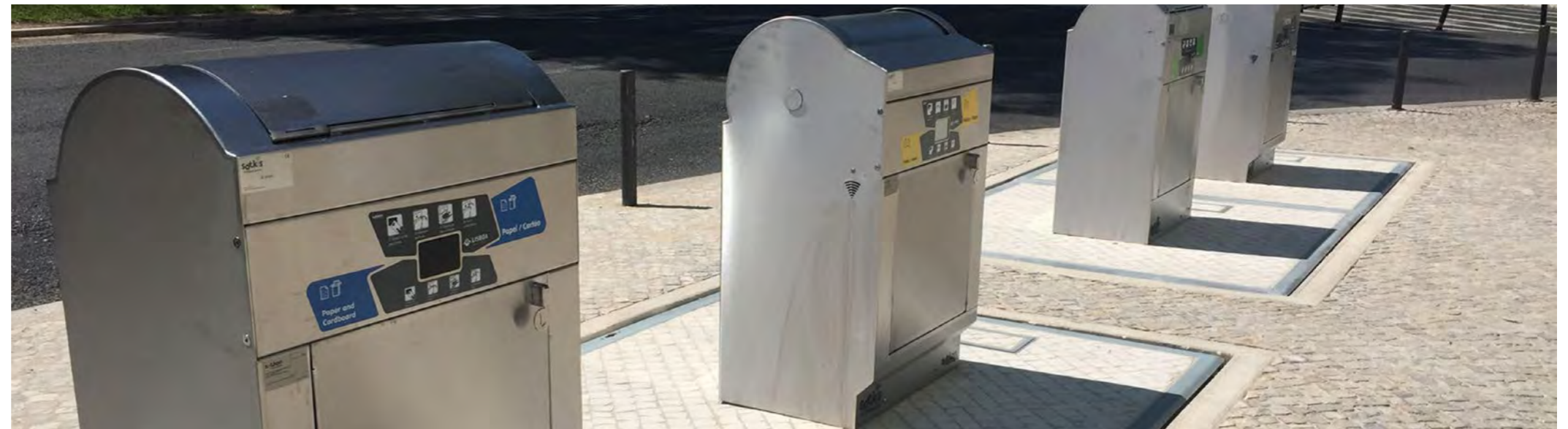
An example of a below ground waste management system with PAYT chip readers and rear access hatches for bulkier waste
