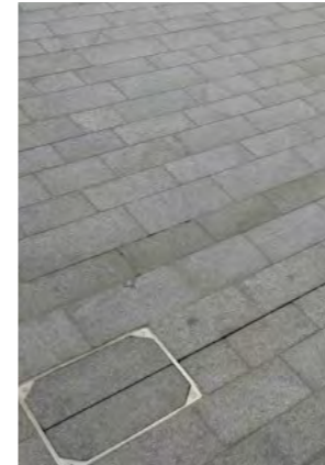
Slot channel maintenance access
