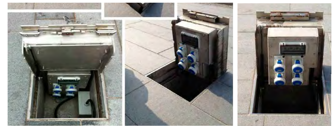
Proposed in-ground power supply points
