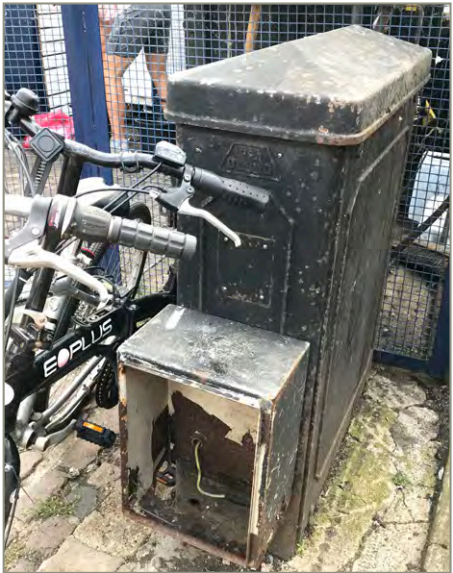
Photos showing existing fuse box for market square.
