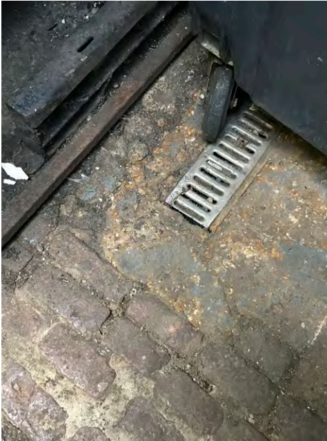
Photo showing existing fat drain
