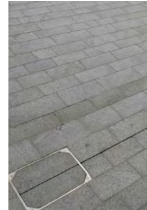
Slot channel maintenance access
