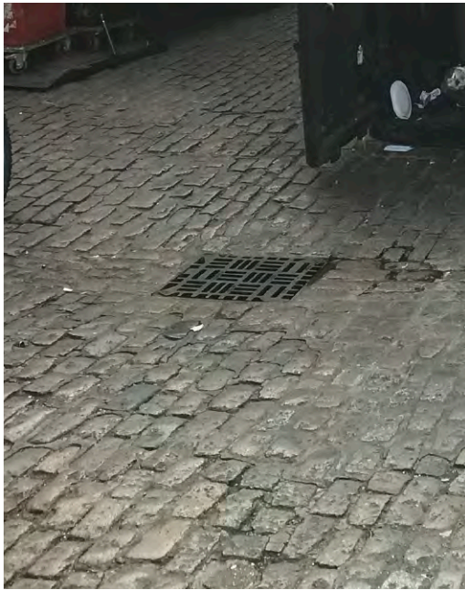
Existing rain gulleys
