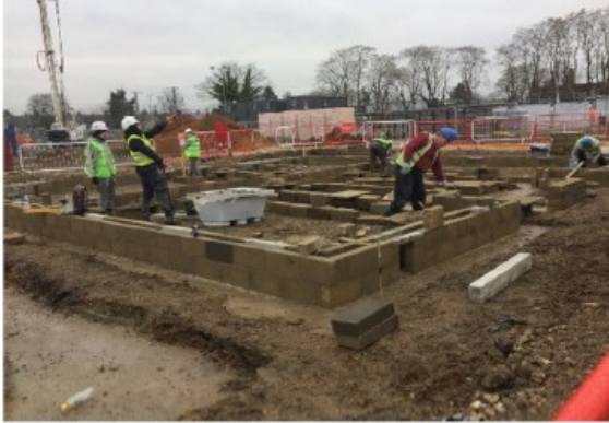
Postal 161 & 162 - Substructure blockwork started
