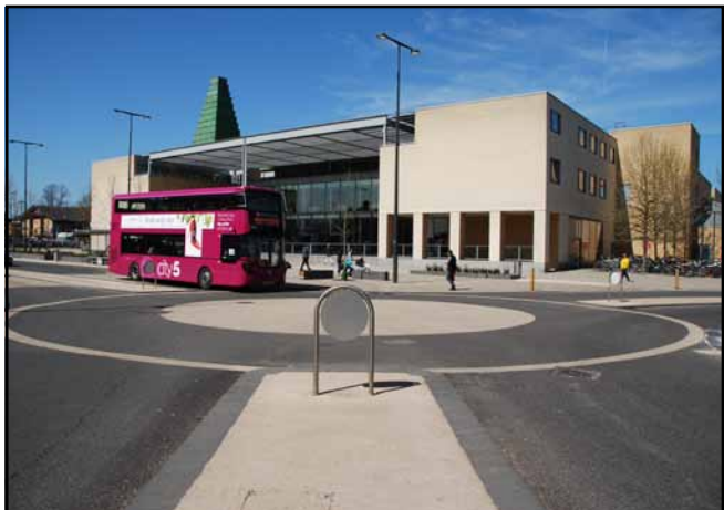
Figure 33: Roundals creates a series of distinct spaces. Median strip (2.5m) separates the direction of vehicle movements, tightens approaches to junctions and provides for informal crossings. Limited signage and road markings encourages lower vehicle speeds (12-15 mph) and assists traffic flows. (Frideswide Square, Oxford).
