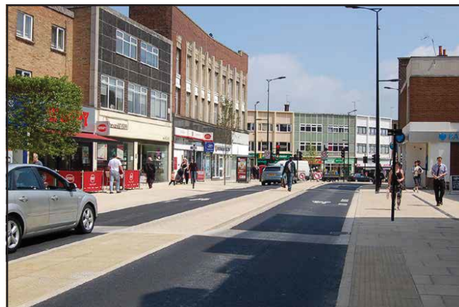
Figure 28: A reduced carriageway width, a central median strip and visual narrowing of the carriageway promotes lower speeds. (Hornchurch, London Borough of Havering).
