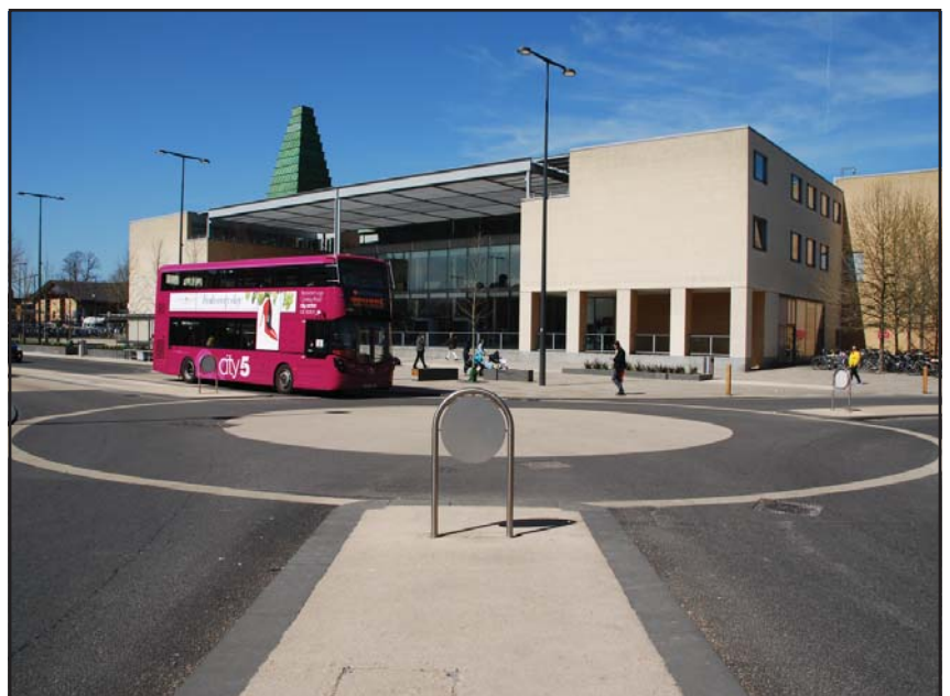
Figure 33: The circular design of roundabouts creates a series of distinct spaces. Generous median strips (2.5m) separate the direction of vehicle movements, tighten vehicle approaches to junctions and provide opportunities for informal crossings. Limited signage and road markings encourages lower vehicle speeds (12-15 mph) and assists traffic flows. (Frideswide Square, Oxford).
