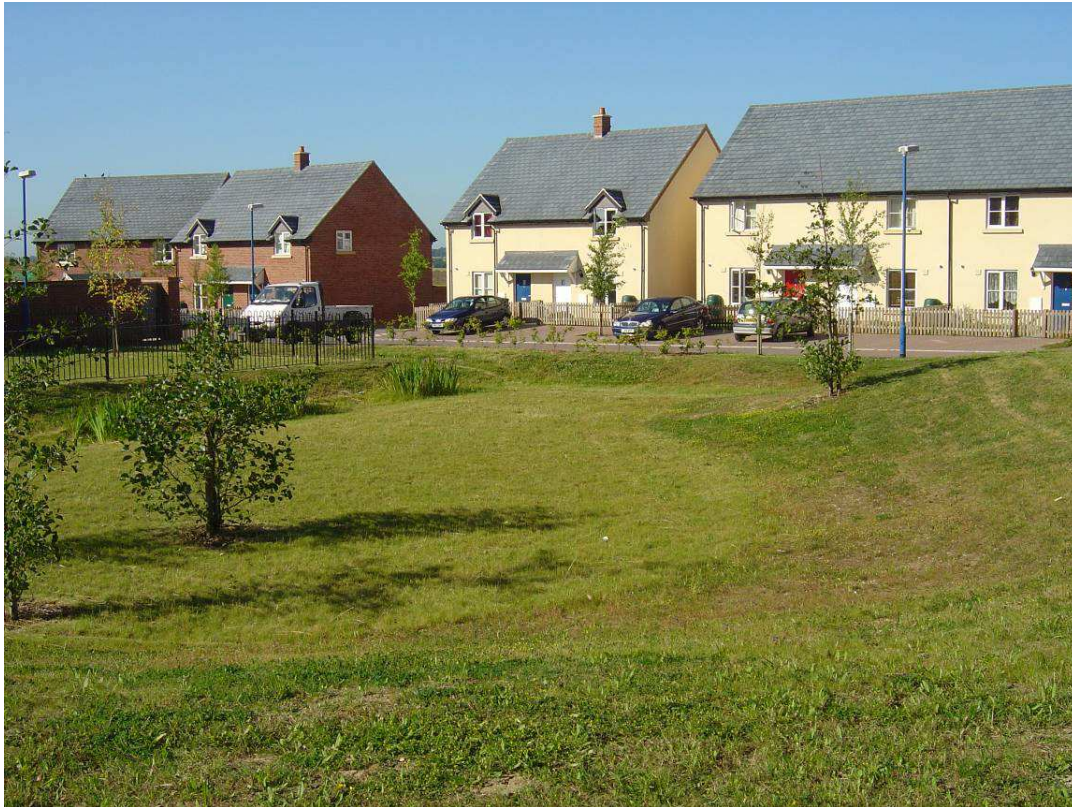
Figure 11 Lamb Drove Sustainable Drainage Scheme
