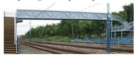
Photo 5 – Typical half-through footbridge with solid parapets (photo from CTS Bridges)
