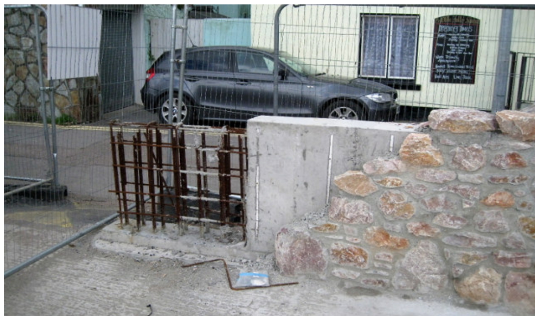
Photo 5.1 - Reinforced concrete flood resistant wall faced with local stone © Robin Stott
