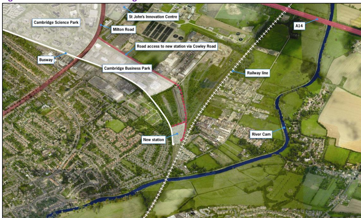
Figure 10: Aerial view of Cambridge Science Park Station.
