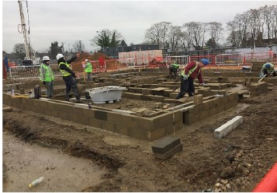
Postal 161 & 162 - Substructure blockwork started
