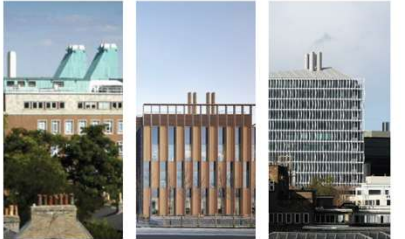
Flue design that reflects innovative spirit of laboratory and respects the historic context. Anglia Ruskin University, Cambridge. Richard Murphy Architects Flues that are integrated into the architectural strategy with high quality architectural expression. Discovery One, Cambridge, HSB Grouped flue articulation St Michael Uten Hub, London. Allies and Morrison
