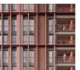
Vertical and horizontal articulation to create visually distinct volumes. Great George Street, Liverpool. Brock Carmichael
