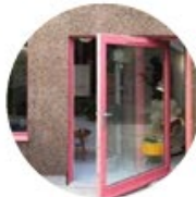
Timber Frames: Clear glazed entrance doors with red coloured frames. Large operable slide and pivot door units.
