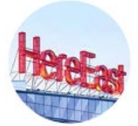
External Signage: Illuminated 3D metal signage in colour to compliment adjacent steel frame.
