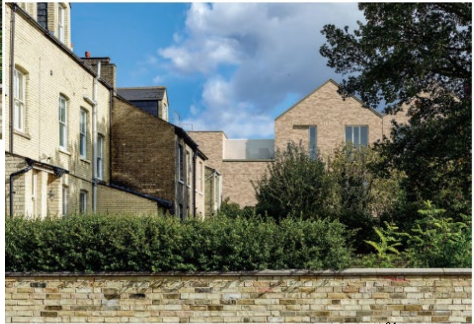
AFTER - View of Block A as seen from Clarendon Road, showing the proposed changes to the roof of Block A to accommodate the ventilation plant required for the revised Net Zero Carbon strategy
