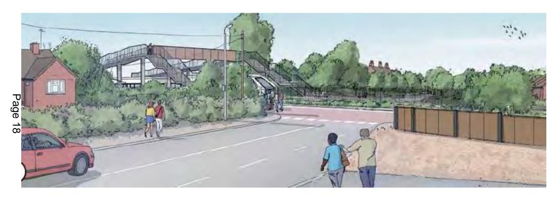
Options 2, 3 and 4 require the Peterborough line level crossing to be removed and replaced with a ramped footbridge structure to maintain connectivity across the railway for pedestrians and cyclists. This illustration shows what the structure could look like.
