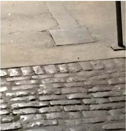
Rotated rectangular setts
