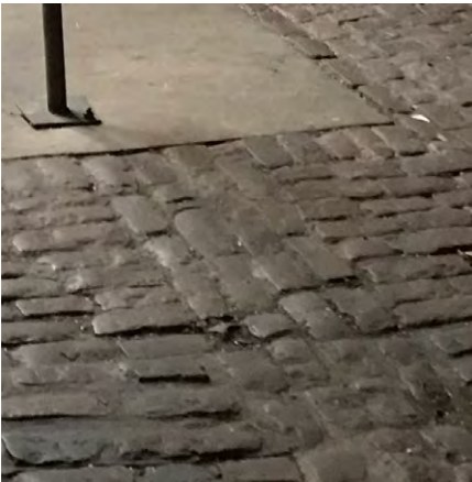
Band of 4 rectangular setts
