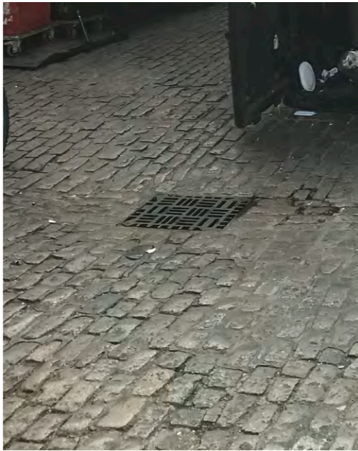
Existing rain gulleys
