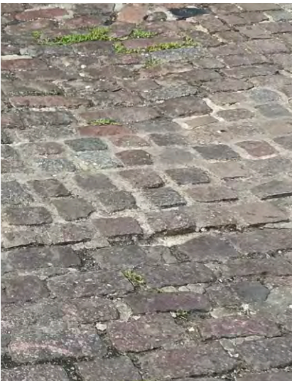
Stack bond (Square setts) limited use
