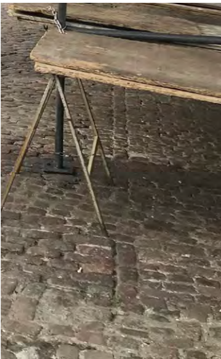
Rectangular sett within square setts
