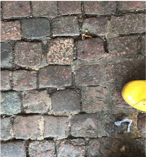
Staggered bond (square setts)
