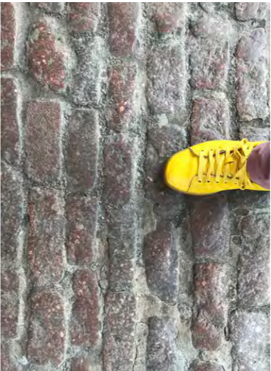
Staggered bond (rectangular setts)
