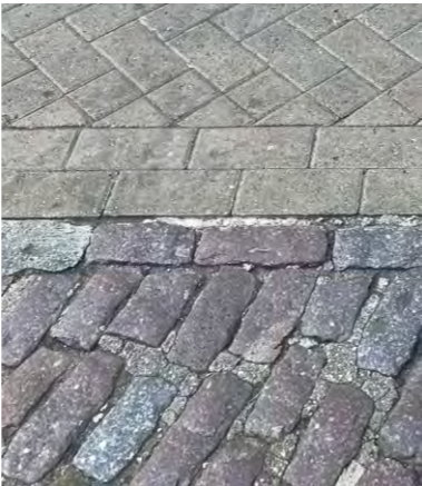
Rotated rectangular setts
